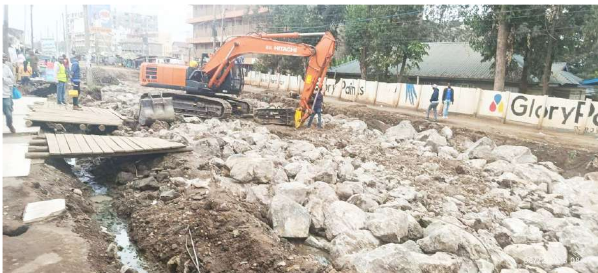
Gataka road construction.
